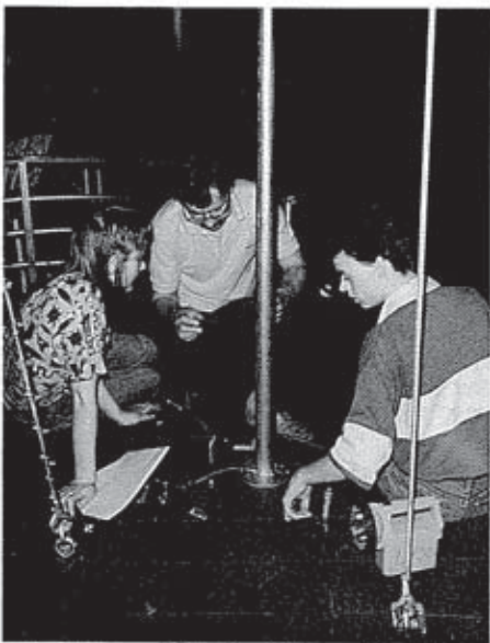
Mike Odam and the electricians get together to deal with a wiring fault.
